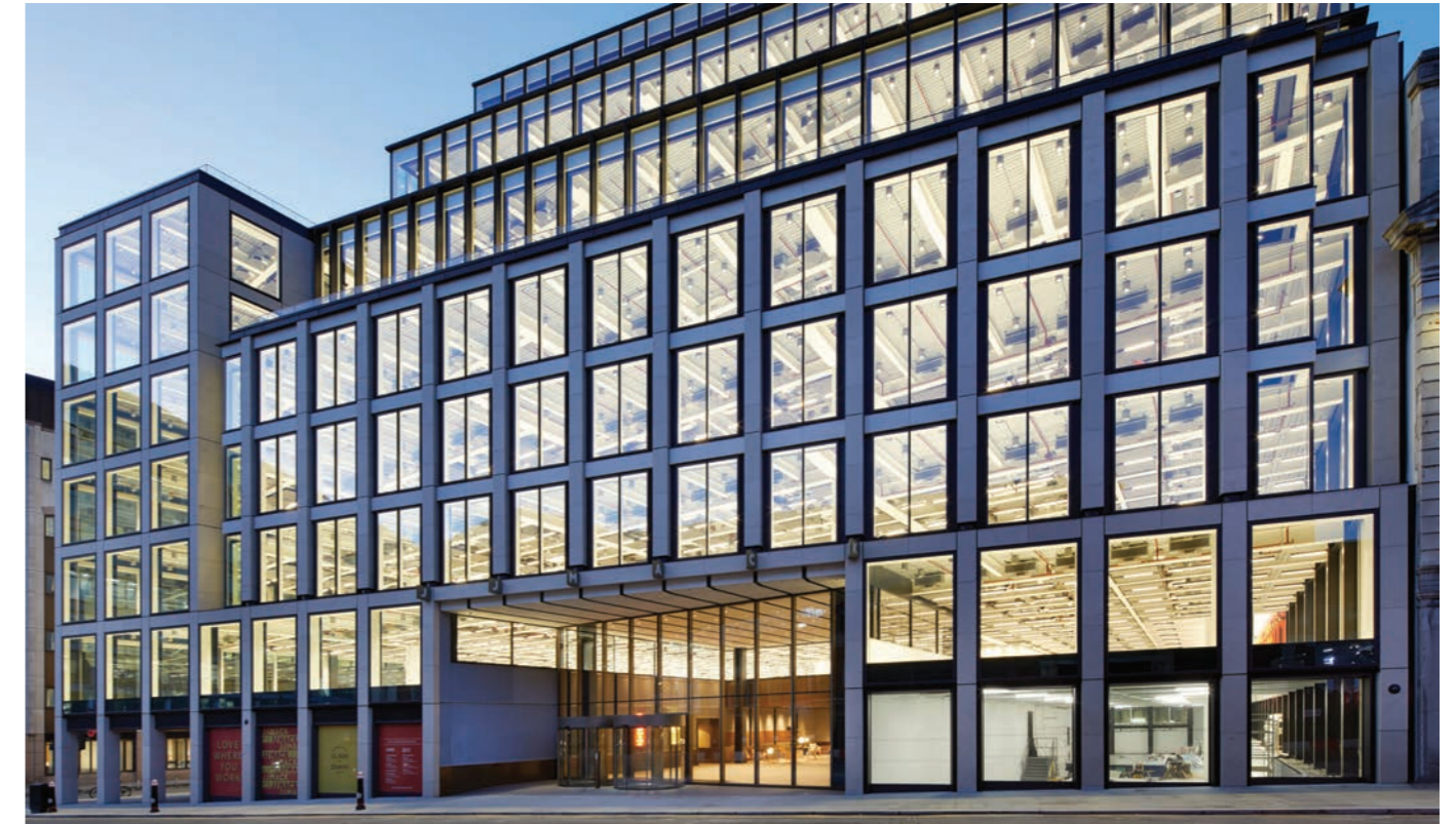
The JJ Mack Building, Farringdon
